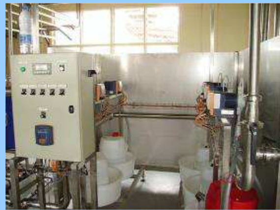
Ozone generator, 4 parameters on line measurement unit, Remineralizing station with 5 solutions
