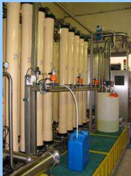
Measure and control devices to manage a global process, ie Ultra Filtration station 80 m 3 /h
