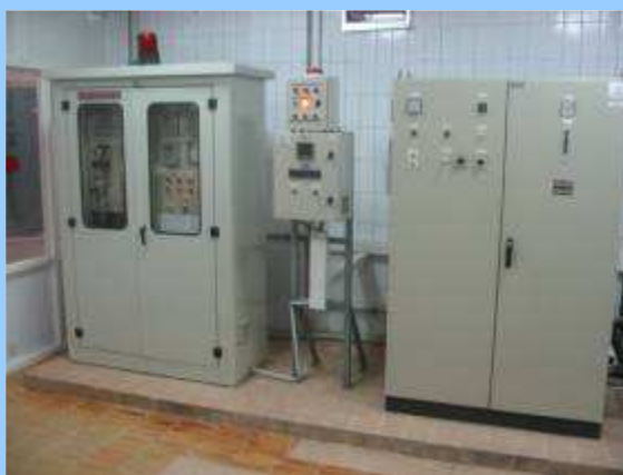
Ozone generator, 4 parameters on line measurement unit, Remineralizing station with 5 solutions
