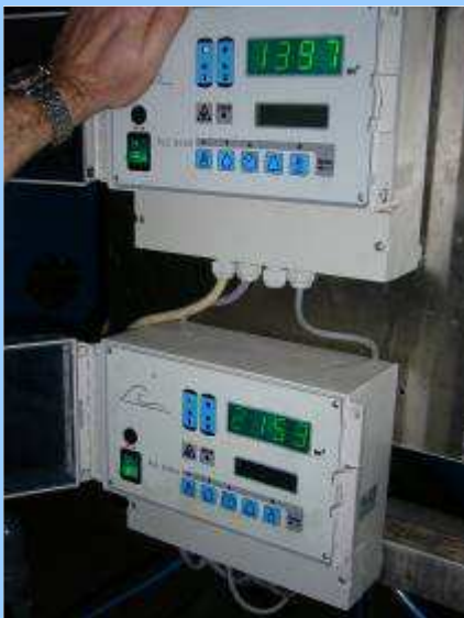
Measure and control devices to manage a global process, ie Ultra Filtration station 80 m 3 /h
