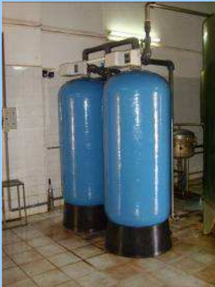
Iron and Manganese removal units 10 and 120 m 3 /h
