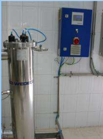
U. V. disinfection units, Process Water 35 m 3 /h and Used Water 1500 m 3 /d
