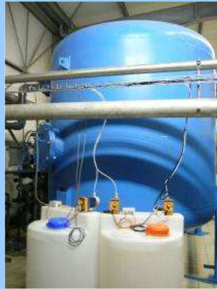
Iron and Manganese removal units 10 and 120 m 3 /h
