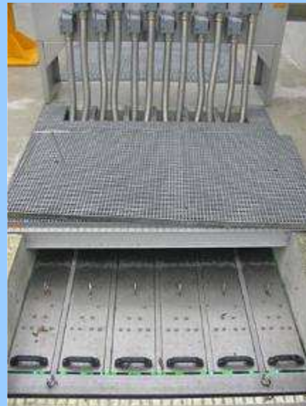
U. V. disinfection units, Process Water 35 m 3 /h and Used Water 1500 m 3 /d
