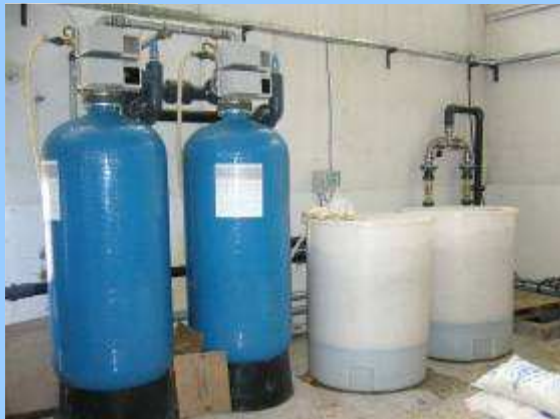
Nitrate removal units with selected ion exchanges resin, 25 and 55 m 3 /h
