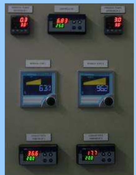
Measure and control devices to manage a global process, ie Ultra Filtration station 80 m 3 /h
